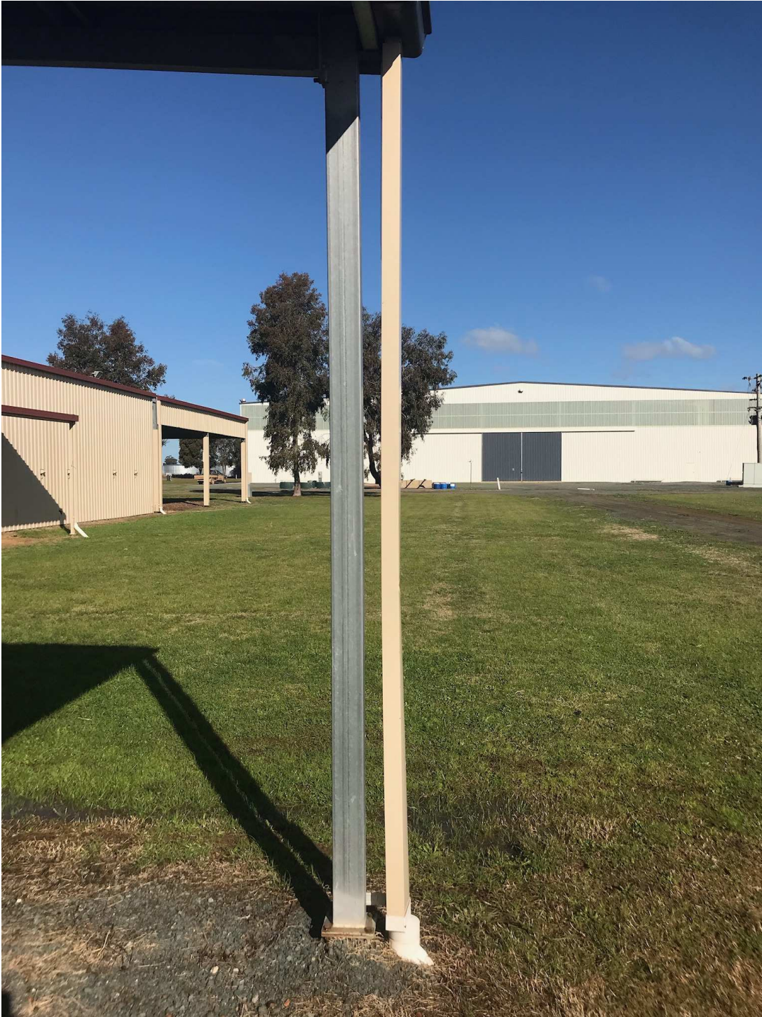
Figure 12: Admin shed post and Satellite antenna area
