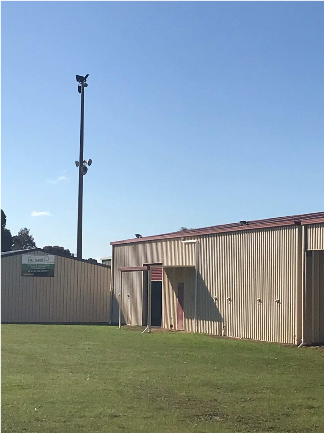
Figure 10: Entrance door(s) and Satellite antenna area - NB GPOs on shed wall
